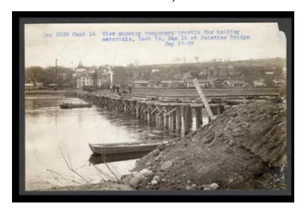
Contract 14. A view showing a temporary trestle for hauling materials at Lock 14, Dam 10 at the Palatine Bridge.
