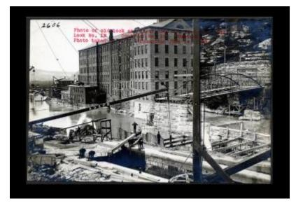
Contract 15. A photo of an old lock and excavation for the east lock wall of Lock 12 in Comstock that was taken by H.J. Richardson.
