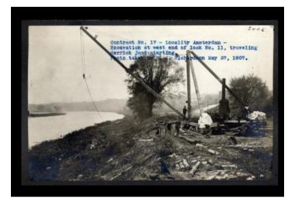
Contract 17. A photo of the excavation at west end of Lock 11 in Amsterdam taken by H.J. Richardson. The photo also shows the traveling derrick just starting.
