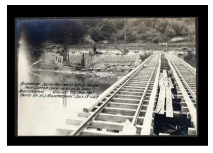
Contract 17. A photo of the excavation of the south abutment and pile driver from the coffer dam head of the south span in Amsterdam taken by H.J. Richardson.
