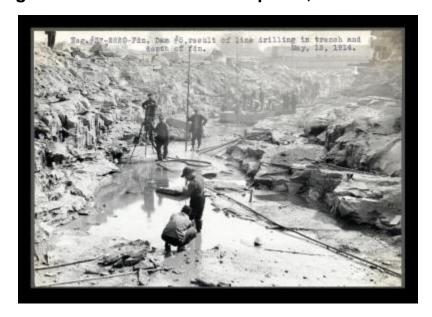
Contract 37. A photo of the foundation of Dam 5, a result of line drilling in trench and depth of foundation.
