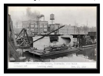
Contract 147. Main-Webster Street Bridge, Tonawanda; pier built. Erecting steel.
