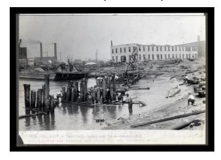
Terminal Contract 19. Greenpoint. Stay lathing and cutting off piles new bulkhead wall.
