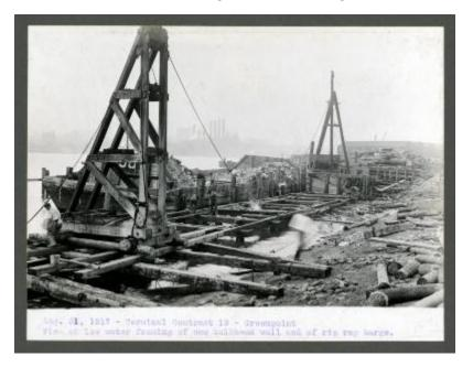
Terminal Contract 19. Greenpoint. View of low water framing of new bulkhead wall and of rip rap barge.
