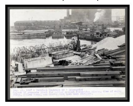
Terminal Contract 19. Greenpoint. Layout of concrete plant for making precast foundation blocks. View of empty forms, filled forms, and blocking that have been striped.
