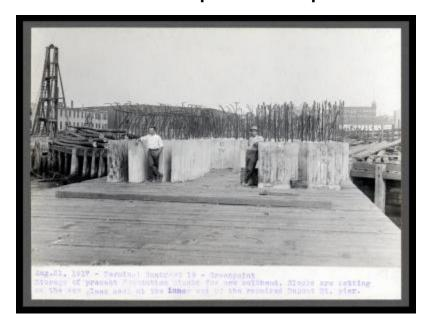
Terminal Contract 19. Greenpoint. Storage of precast foundation blocks for the new bulkhead. Blocks are sitting on the new plank deck at the inner end of the repaired Dupont Street pier.
