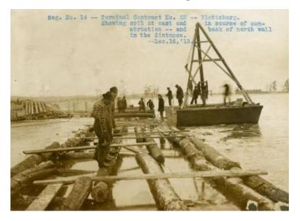
Terminal Contract 23. Plattsburgh. Showing crib at east end in course of construction--and back of north wall in the distance.
