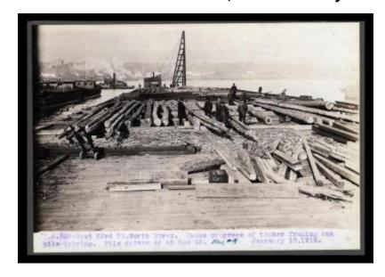
Terminal Contract 38. West 53rd Street. North River. Shows progress of timber framing and pile driving. Pile driver is at Row 65.
