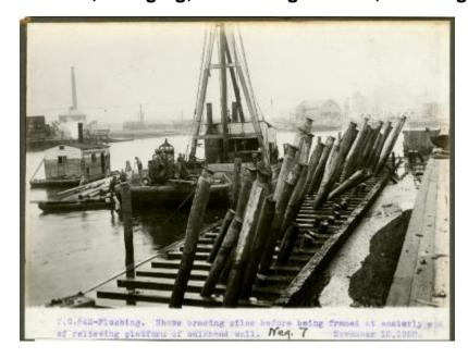
Terminal Contract 43. Flushing. Shows bracing piles before being framed at easterly end of relieving platform of bulkhead wall.
