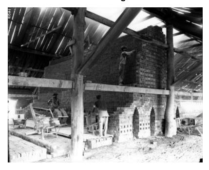
Building a brick kiln, showing arches for fires and method of arranging brick as part of the brickmaking process. Haverstraw, NY, (1912).
