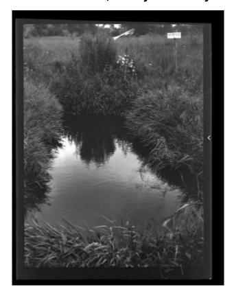
This old waterhole, constructed in 1933, doesn't meet the standards of the 1936 Civilian Conservation Corps. The hole will need to be expanded, cleaned, and lined with stone. Once this is done, the waterhole will aid fire suppression in this forest in Schuyler County. This image was created to record the reforestation work of the Civilian Conservation Corps under the supervision of the New York State Conservation Department.
