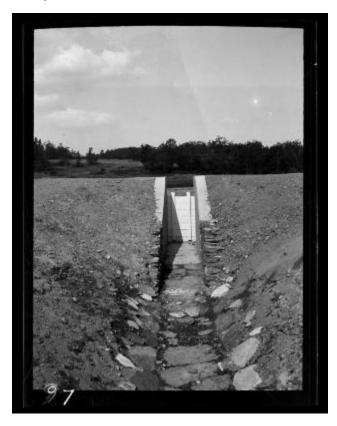
This is the sluice gate for the overflow spillway built for the expanded Palmer Pond by the Civilian Conservation Corps. CCC camp S-92, stationed in Almond, has been damming and expanding the pond for recreational use. This image was created to record the reforestation work of the Civilian Conservation Corps under the supervision of the New York State Conservation Department.
