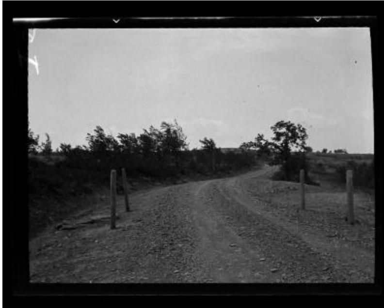
This truck trail, culvert and set of guard posts are the work of the Civilian Conservation Corps. This trail was likely constructed to improve access to a reforestation area and to assist with firefighting efforts. This trail, #202-1, is the work of CCC camp S-123, stationed in Beaver Dams, N.Y. This image was created to record the reforestation work of the Civilian Conservation Corps under the supervision of the New York State Conservation Department.
