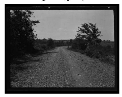
This truck trail, and the set of guard posts in the distance, is the work of the Civilian Conservation Corps. This trail was likely constructed to improve access to a reforestation area and to assist with firefighting efforts. This trail, #202-1, is the work of CCC camp S-123, stationed in Beaver Dams, N.Y. This image was created to record the reforestation work of the Civilian Conservation Corps under the supervision of the New York State Conservation Department.
