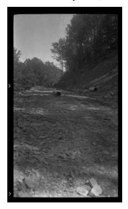
A truck trail is under construction by the Civilian Conservation Corps, camp S-118, stationed in Truxton, N.Y. The road has been leveled and gravel laid down. Large pipes lay in the road, perhaps scheduled to become a culvert. These roads were constructed by the CCC to aid in their reforestation and fire suppression projects. This image was created to record the reforestation work of the Civilian Conservation Corps under the supervision of the New York State Conservation Department.
