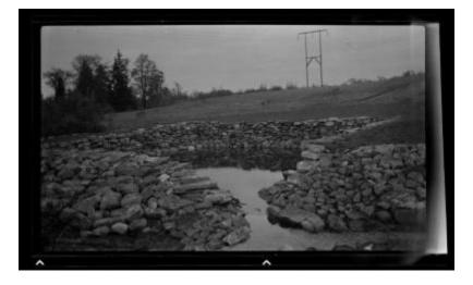
This waterhole is a production of the Civilian Conservation Corps, camp S-134, stationed in Canton, N.Y. The crew excavated a hole and lined it with stone to form a receptacle for water drawn from the brook. It will serve as a source of water during firefighting efforts. This image was created to record the reforestation work of the Civilian Conservation Corps under the supervision of the New York State Conservation Department.
