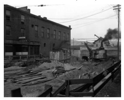
A view of Fifth Street looking east on street excavation. The excavation was necessary for passing underneath the railroad overpass. This photograph was taken to document the progress of construction.
