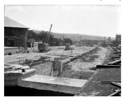
Construction of two elevated Lackawanna tracks that would be on either side of the passenger station's central boarding platform. This photograph was taken to document the progress of construction.
