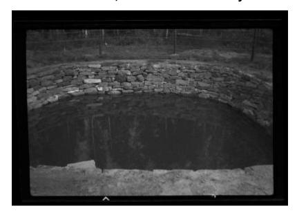
This waterhole was constructed by the Civilian Conservation Corps, camp S-95, stationed in Brasher Falls. The crew excavated a hole and lined it with stone to form a receptacle for water drawn from a spring. It will serve as a source of water during firefighting efforts. This image was created to record the reforestation work of the Civilian Conservation Corps under the supervision of the New York State Conservation Department.
