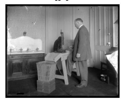
View of a man demonstrating the operation of a "trout tagging machine." He is holding a trout, and is about to stamp a mark on its tail. There is a basket next to the machine that he appears to be tossing fish into. The date and location are unknown, but it is probably ca. 1918-1920. This image was created to record the game fish hatchery activities of the New York State Conservation Commission.
