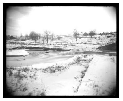
View of a dam on Caroga Creek near Rosewood in Ephratah, Fulton County in winter. The dam was owned by the Rockwood Manufacturing Company, and caused erosion of the stream bank and the stone paving. This image was created to record the waterpower activities of the New York State Conservation Commission.
