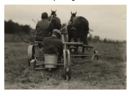
Two men seated in the Champion Duplex Reforesting Machine. The machine was invented by the Champion Sheet Metal Company, of Cortland, N.Y. The machine was built to carry two men and pulled by a tractor over plowed land; it was mainly used to reforest former farm land. Photograph was taken in a field in western New York, near the College of Environmental Science and Forestry at Syracuse.
