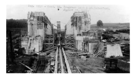
Contract 11. A photo of the construction of Erie Canal Lock 5 in Waterford, N.Y. that was taken on August 20, 1908.
