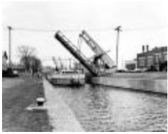
Barge Canal. Day Peckinpaugh Passing Lift Gate (NYSA_A0834-77_004)
