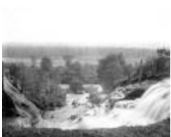
Water rushes through a break in the Forestport Feeder canal levee, 1899 (NYSA_A0834-77_B5_F11)
