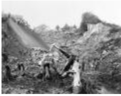
Break in canal at Forestport, N.Y. (NYSA_A0834-77_B5_F12)
