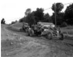
Highway construction at Haines Falls, Hunter, NY (NYSA_17672-92_B39_6386_7)
