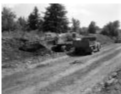
Highway construction at Haines Falls, Hunter, NY (NYSA_17672-92_B39_6386_5)
