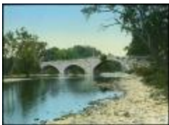
Old Stone Bridge over the Catskill Creek (NYS A3045_10646)
