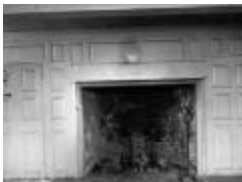
Fireplace in the house of Dirk Van Veghten in Old Ford on Catskill Creek (NYS A_0245-77_Greene_B04_44)
