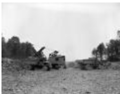
Catskill Thruway progress photograph (NYS 17672-92_B30_4511_7)
