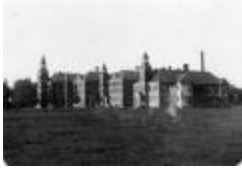
Mental Health Custodial Facilities. Lincoln State School Main Building (NYS_A4228-78_B1_F9_405)
