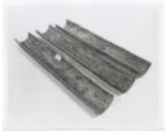
Belmont Lake State Park, Corroded Irrigation Pipes (NYSA_B2877-22_P_B3_F111_003)
