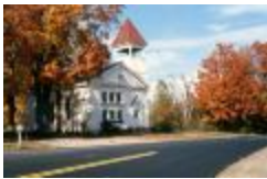
Porter Corners Methodist Church in Saratoga County (NYSA_19125-07_B5_SL29696)
