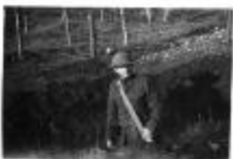
Man in Trench 2 (NYSA_A0412-78_B09_F10_Man_trench)
