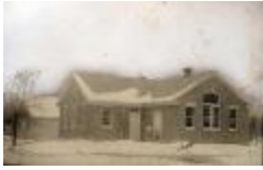
Thomas Indian School Photograph. Exterior View of Laundry Building and Vegetable Cellar (NYSA_A1913-77_37)
