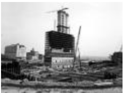
Progress Photo. Construction of Corning Tower. (NYSA_15727_B4_002)
