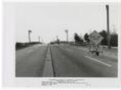
Improvements to bridges (NYSA_B2877-22_P_B1_F16_016)
