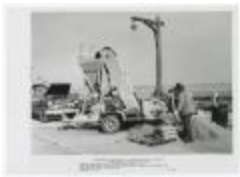
Improvements to bridges (NYSA_B2877-22_P_B1_F16_004)
