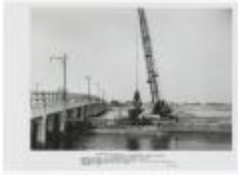
Improvements to bridges (NYSA_B2877-22_P_B1_F16_012)
