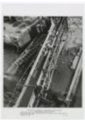
Improvements to bridges (NYSA_B2877-22_P_B1_F16_008)
