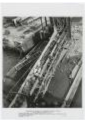
Improvements to bridges (NYSA_B2877-22_P_B1_F16_010)
