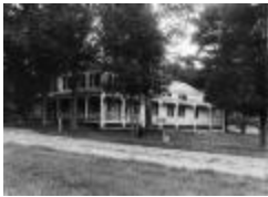
Dowling House in Lake George, New York (NYSA_A0245-77_Warren_B21_44)
