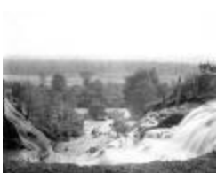
Water rushes through a break in the Forestport Feeder canal levee, 1899 (NYSA_A0834-77_B5_F11)
