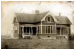
Thomas Indian School Photograph. Exterior View of Hospital Building (NYSA_A1913-77_14)
