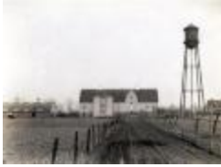
Thomas Indian School. View of Entrance to Farm Buildings and Water Tower (NYSA_A1913-77_39)
