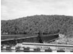
Spiers Falls Power Dam in Glens Falls, New York, 1938 (NYSA_A0245-77_Warren_B21_63)
