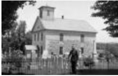
Fort Herkimer Church with Abbot Livingston Marshal in Herkimer, New York. 1938 (NYSA_A0245-77_Herkimer_B04_63)
