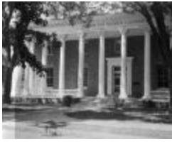
Headquarters of the New York State Historical Association in Cooperstown, New York. October 15, 1941 (NYSA_A0245-77_Otsego_B11_67)
