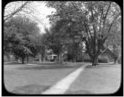
River front mansion with servants house near Fredericksburg, Virginia (NYS_A3045-78_X_10192)
