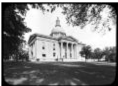
Ontario County Courthouse, Canandaigua (NYS A3045-78_X_3117)
