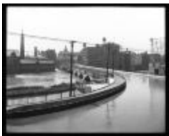
Erie canal aqueduct near Genesee River, Rochester (NYS A3045-78_X_3118)
