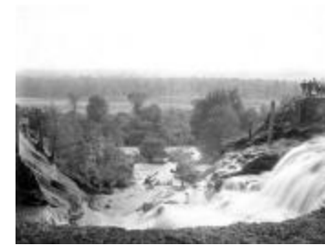
Water rushes through a break in the Forestport Feeder canal levee, 1899 (NYSA_A0834-77_B5_F11)
