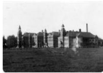
Mental Health Custodial Facilities. Lincoln State School Main Building (NYSA_A4228-78_B1_F9_405)
