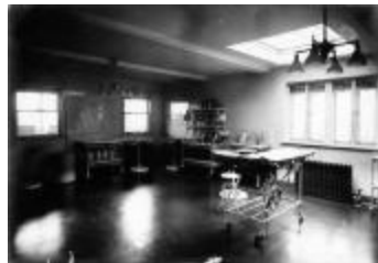
Mental Health Custodial Facilities. Vineland State Home. Operating Room (NYSA_A1994-77_B1_F7_P114)
