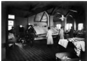
Mental Health Custodial Facilities. Syracuse Custodial Facility. Mangle Machine (NYSA_A1994-77_B3_F2_P13)
