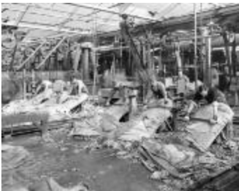
Tanning: Beam Workers at Endicott Johnson Plant. (NYS A_3045-78_A9965)
