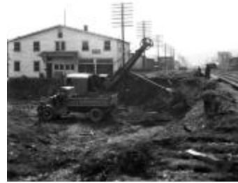
Railroad project, Nanticoke Avenue, Endicott, NY (NYSA_17672-92_B12_1105_001)
