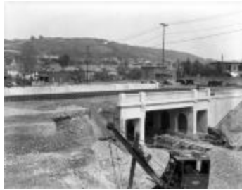
Railroad project, Binghamton, NY (NYSA_17672-92_B12_1298_001)
