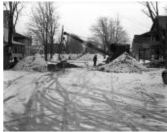
Railroad project, Nanticoke Avenue, Endicott, NY (NYSA_17672-92_B11_1093_001)
