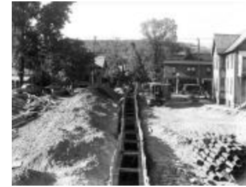
Railroad project, Nanticoke Avenue, Endicott, NY (NYSA_17672-92_B12_1247_001)
