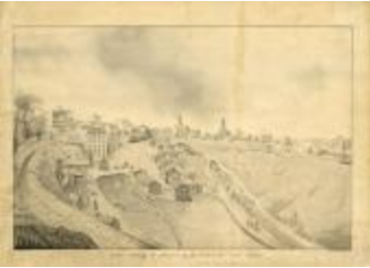
View Showing the Progress of the Work on the Lock Section (NYSA_B0379-85_V17_09- 01-1839)
