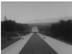
Opening of the Tappan Zee Bridge on the New York Thruway, 1955 (NYSA_14512-91_mpf16_1955-12-15a)
