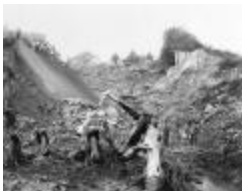
Break in canal at Forestport, N.Y. (NYSA_A0834-77_B5_F12)
