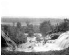
Water rushes through a break in the Forestport Feeder canal levee, 1899 (NYSA_A0834-77_B5_F11)
