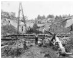
Break in Canal at Forestport, N.Y. (NYS A0834-77_B5_F14_Forestport2)
