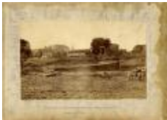
Condition of the work on the new Capitol at Albany, N.Y., photograph A (NYS A1897-78_A)
