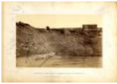
Condition of the work on the new Capitol at Albany, N.Y., photograph B (NYS A1897-78_B)
