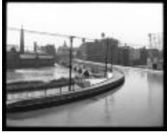
Erie canal aqueduct near Genesee River, Rochester (NYSA_A3045-78_X_3118)
