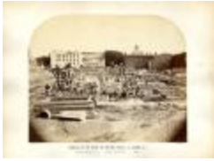
Condition of the work on the new capitol at Albany, N.Y. (NYSA_B0701-85_B2_F06)
