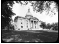
Ontario County Courthouse, Canandaigua (NYSA_A3045-78_X_3117)
