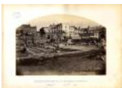
Condition of the work on the new Capitol at Albany, N.Y., photograph 10 (NYS_A1897-78_10)
