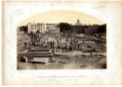
Condition of the work on the new Capitol at Albany, N.Y., photograph 11 (NYS A1897-78_11)
