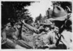
Men in Trench (NYSA_A0412-78_B09_F10_Men_trench)
