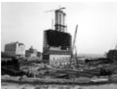
Progress Photo. Construction of Corning Tower. (NYSA_15727_B4_002)
