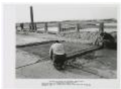
Improvements to bridges (NYSA_B2877-22_P_B1_F16_014)
