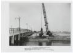
Improvements to bridges (NYSA_B2877-22_P_B1_F16_012)
