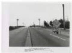
Improvements to bridges (NYSA_B2877-22_P_B1_F16_016)
