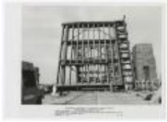
Improvements to bridges (NYSA_B2877-22_P_B1_F16_002)
