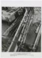
Improvements to bridges (NYSA_B2877-22_P_B1_F16_008)
